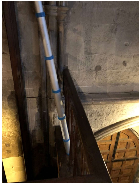
The west access to the south side of the organ. The gallery extension, height of the gallery from the floor, and the angle and method of placing a ladder over the staircase can all be seen. Ascending this ladder would effectively place the tuner over the drop to the floor
