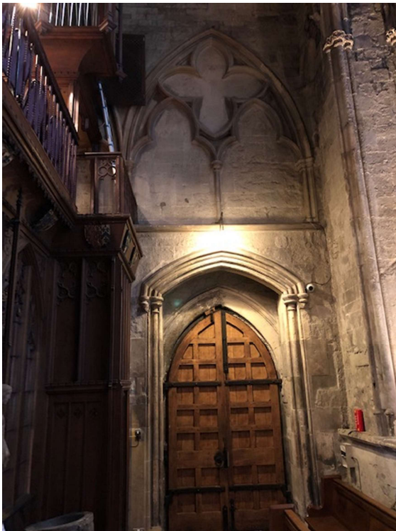
The west access to the south side of the organ. The gallery extension, height of the gallery from the floor, and the angle and method of placing a ladder over the staircase can all be seen. Ascending this ladder would effectively place the tuner over the drop to the floor
