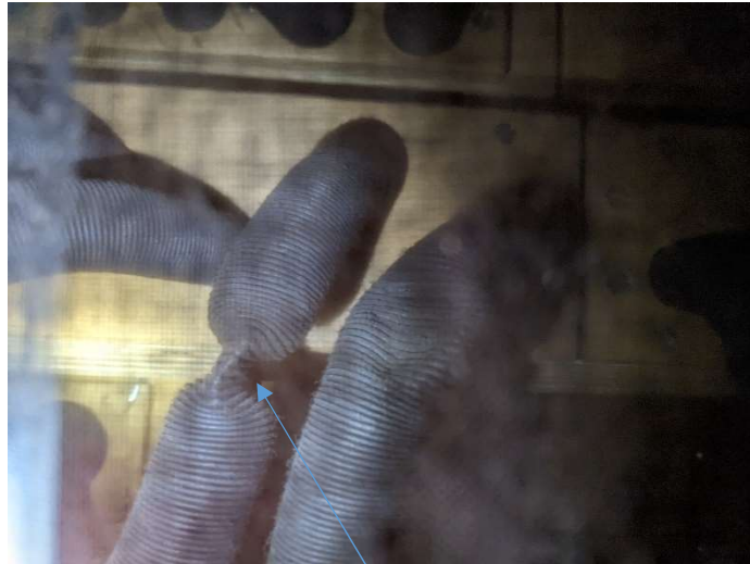
Example of constricted copex conveyance reducing wind supply to a pipe
